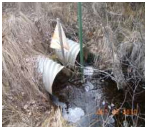
Figure 2 – Downstream End Unnamed Trib to Filson at Spruce Rd Note: free discharge and magnitude of discharge << 1 cfs
