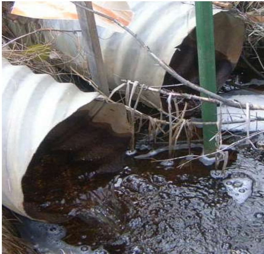
Figure 3. Exploded view of downstream end of Spruce Road culverts
